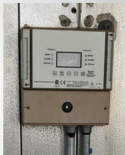
The ConsoliDator+ replaced this old degraded controller. The small display is hardly readable and it is exposed to the outside elements.
