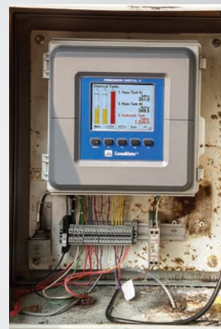
Enclosure opened showing wiring to ConsoliDator+
