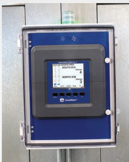
The ConsoliDator+ is fully protected from the elements by a PDA3939 NEMA 4X plastic enclosure that includes a clear front door for easy access.
