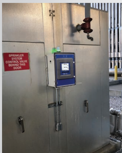
The ConsoliDator+ PD9000 was installed near the ammonia tank on the outside panel of the sprinkler system.
